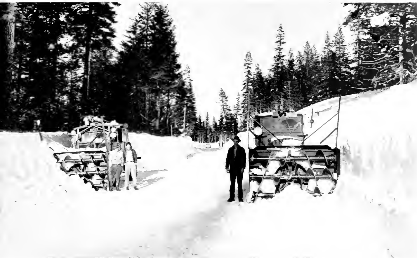
Close-up view of two of the rotary snow plows engaged in widening operations in the Donner Summit area
